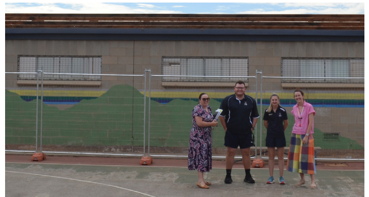
DEVELOPMENT: If only the walls could talk! The old change rooms at Bosco Campus were demolished to make way for future projects. Pictured are staff (and Old Scholars) Mrs Katie Pole (Keane-1995), Mr Caleb Brown (2013), Miss Talia Phillippis (2018) and Mrs Annie Olsen (Richter-2004)
